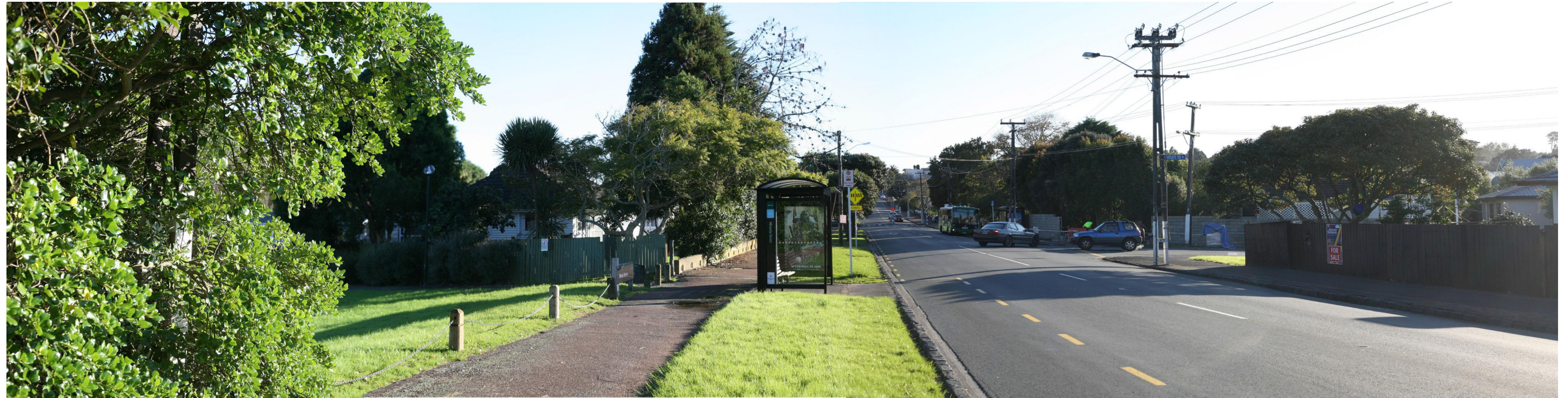
View from Blockhouse Bay Road looking North
